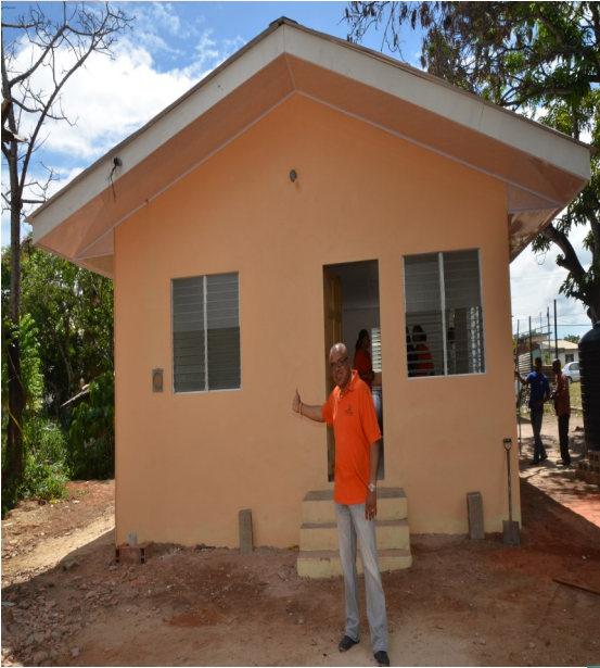
Photo above Mr. Surujdeo Mangaroo, Chairman of NCSHL stands in front of Mr. Curtis Garcia home in Bypass Arima. NCSHL signed a MOU with the MIC for the construction of this starter home.
